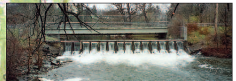
Otsego Lake levels have been partially managed in recent times by the dam located by Bassett Hospital which limits flooding and conserves summer water levels while posing some issues for shoreline stability.
