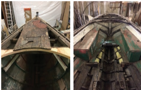
With deck removed during restoration.
